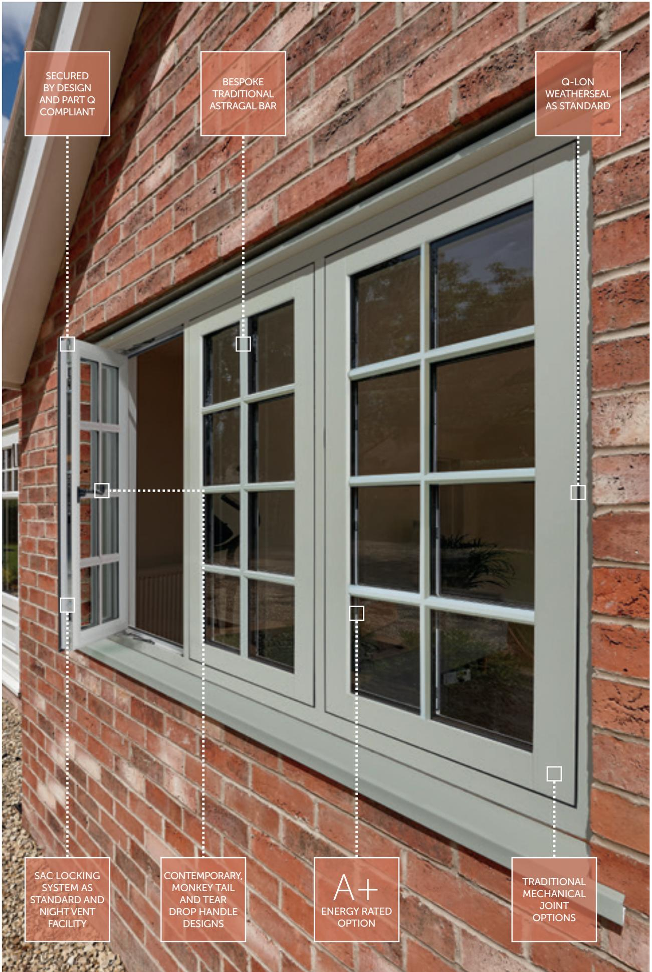
SECURED BY DESIGN AND PART Q COMPLIANT
